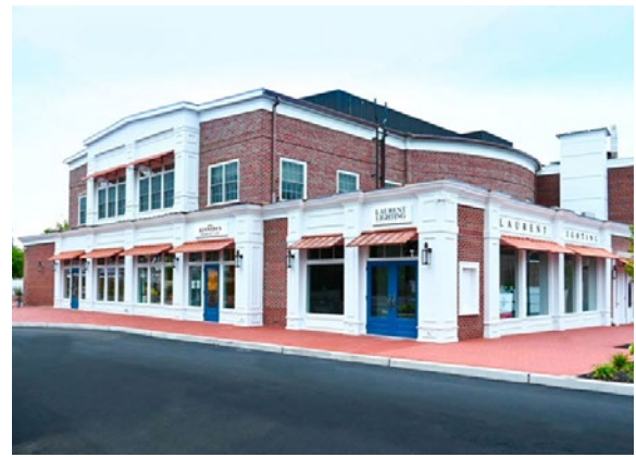
▲ The 1927 Darien Playhouse at 1077 Boston Post Road was an adaptive reuse project that repurposed the structure as a mixed-use property (photo by V20 Group, LLC)
