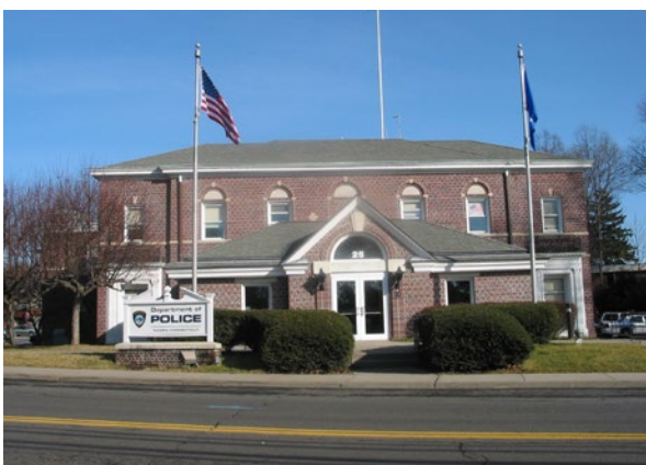
▲ The Police Department building (photo courtesy of the Department of Planning & Zoning)
