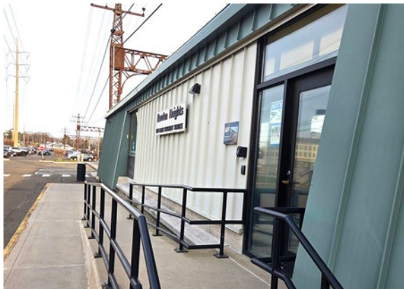
▲ The Noroton Heights train station building in 2026. An ADA-compliant handicap ramp was added in 2018 as part of a broader CTDOT platform replacement project.
