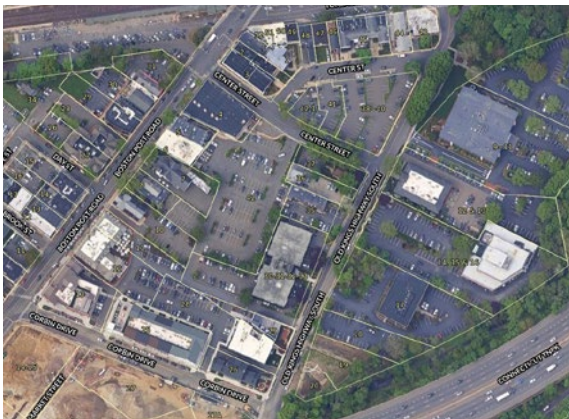
▲ Aerial photo from the Town's MapGeo showing properties forming the block around Boston Post Road, Old King's Highway South, Center Street, and Corbin Drive
