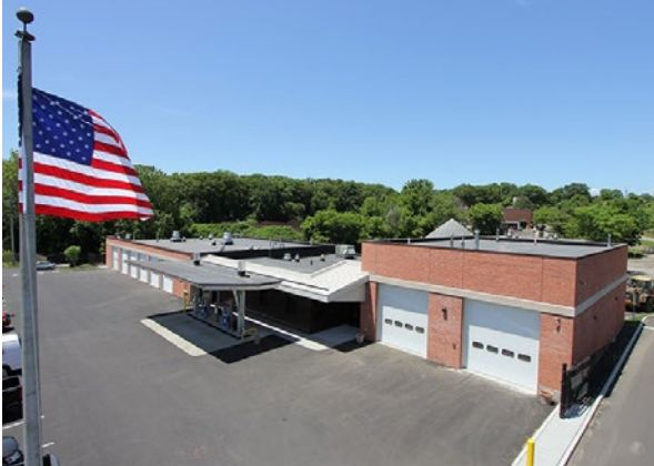
▲ The DPW Garage (photo courtesy of the Department of Public Works)
