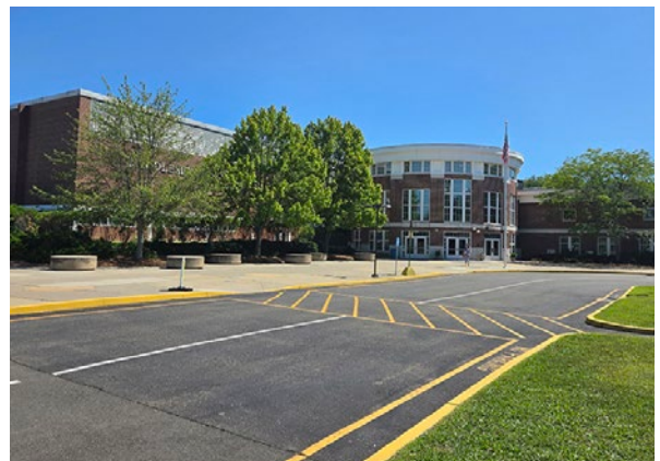
▲ Middlesex Middle School, located along Hollow Tree Road north of the Noroton Heights train station
