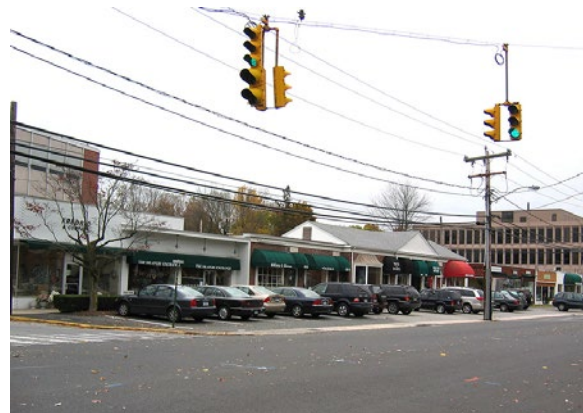
▲ The old "Fairbanks Block," or the south side of Boston Post Road between Exit 11 and Corbin Drive (photo courtesy of the Planning & Zoning Department)
