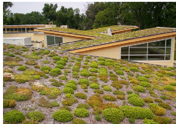
▲ An example of a green roof (photo by Arlington County, VA, licensed by CC BY-SA 2.0)
