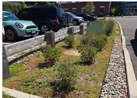
▲ Green stormwater infrastructure in the parking lot of Ox Ridge Elementary School in the form of a rain garden
