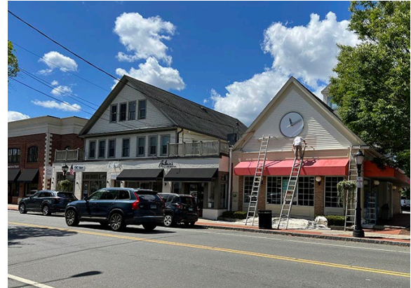
▲ Buildings in the Central Business District (CBD) zone along Boston Post Road
