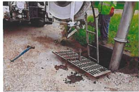
▲ Cleaning out catch basins is important to ensure proper drainage (photo by Mr G's Excavation & Grading, licensed by CC BY-NC 4.0)
