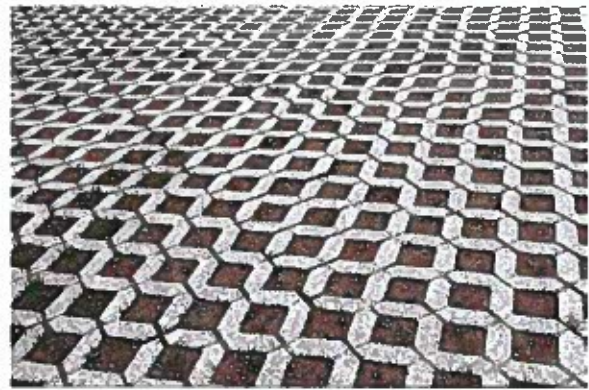
▲ A driveway made of permeable pavers, which, when maintained properly, reduce stormwater runoff by allowing it to infiltrate the soil
