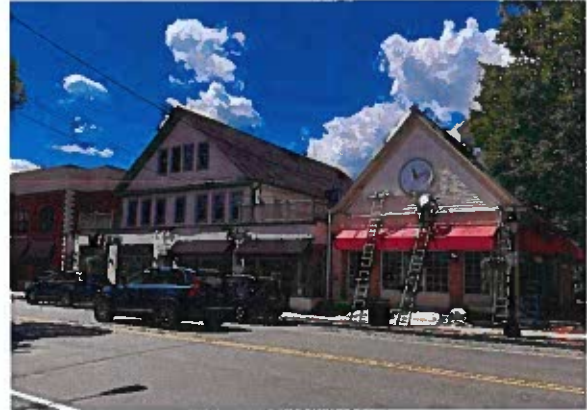
▲ Buildings in the Central Business District (CBD) zone along Boston Post Road
