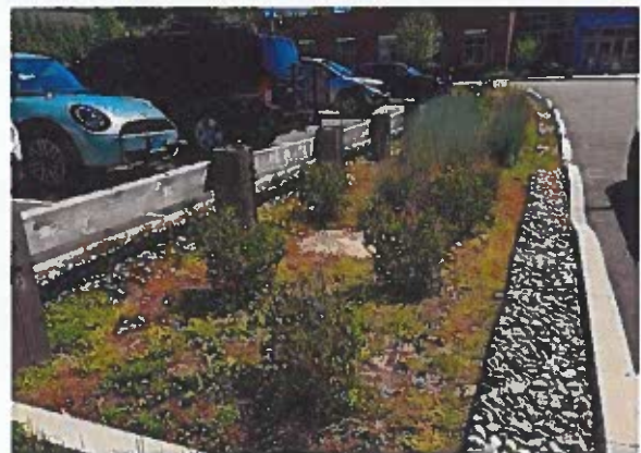
▲ Green stormwater infrastructure in the parking lot of Ox Ridge Elementary School in the form of a rain garden
