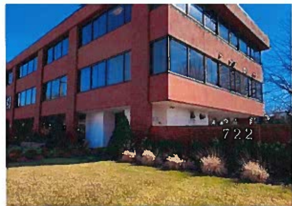
▲ A medical office building in the Designed Business (DB) zone along Boston Post Road
